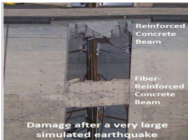
Figure 5.1 Crack pattern in with and without steel fiber concrete
